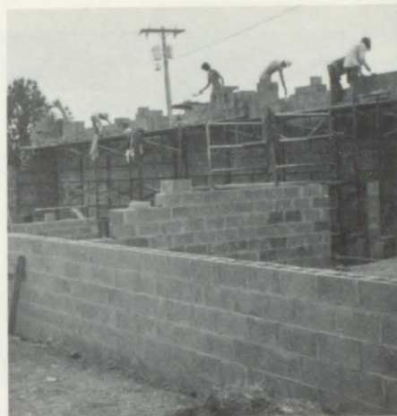
Masonry class builds new Viking baseball home in Haynesfield Park.
