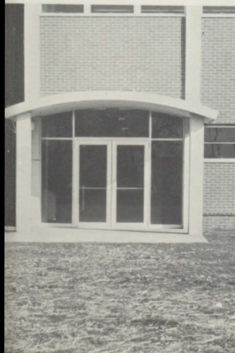
Entrance to the new wing.
