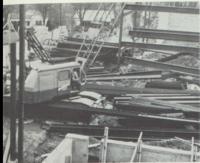
Putting up the steel.
