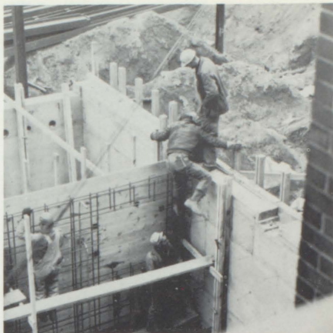
Making forms for the new boiler room.
