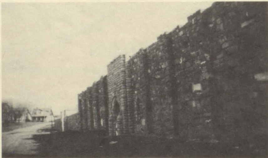
STADIUM - UNDER CONSTRUCTION
